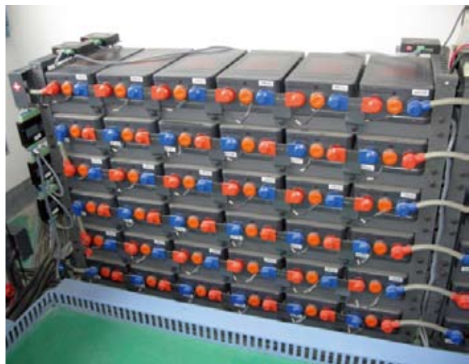
Onsite Wire Connection
